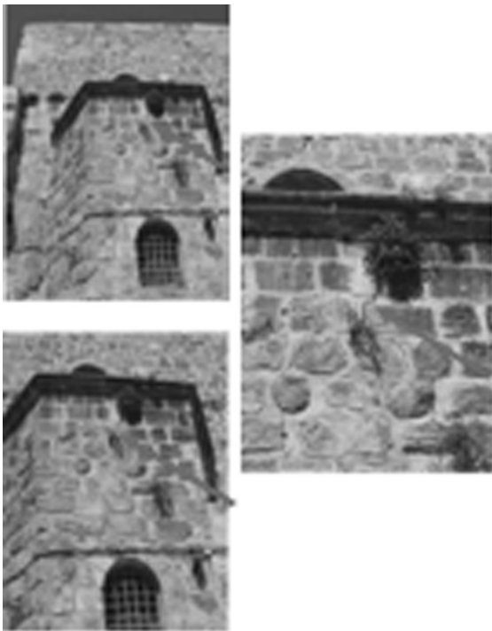
Figure 3.24 Pre-existing cracks in the masonry of the wall of the Church of the Holy Sepulchre enlarged by the earthquake of 11 February 2004 in the northeast of the Dead Sea ( M_s 5.0) (A. Salamon).
