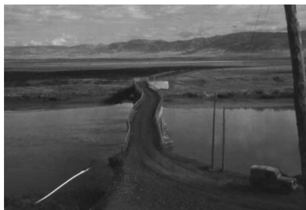
Figure 3.44 The stone-masonry bridge on the Murat Nehri (Euphrates), at an epicentral distance of 40 km, photographed after the Varto earthquake of 19 September 1966 ( M_s 6.8).
