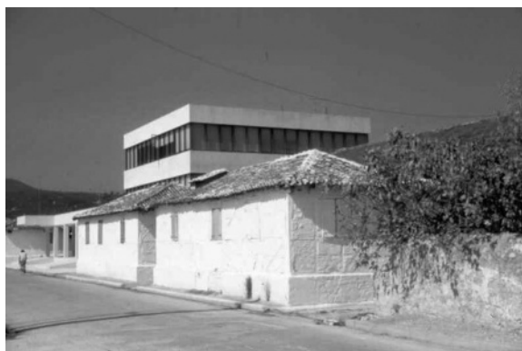
Figure 3.35 In the foreground can be seen two of the few remaining timber-reinforced, single-storey houses in Leukas, built with a method of construction introduced by carpenters of the British Navy after the destructive earthquake of 19 January 1825.
