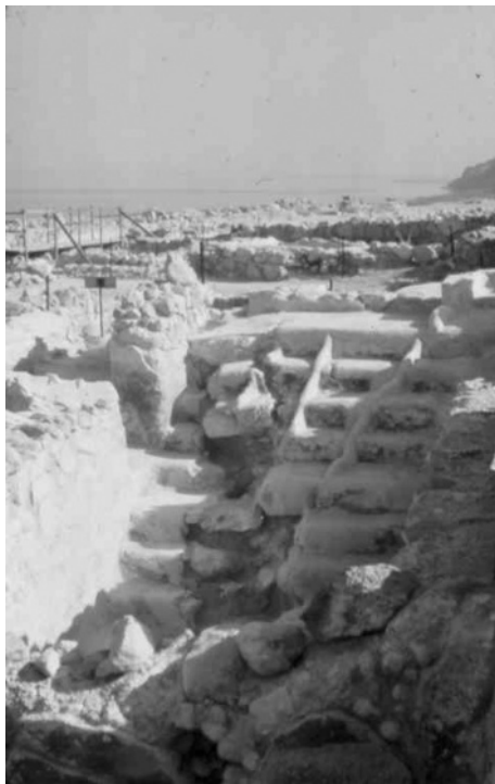
Figure 3.2 Originally, a crack that cuts through the steps down to the water cistern at Qumran was attributed to surface faulting in the earthquake of 31 BC. Recent conservation work established that the shearing off of the steps was the result of differential settlement of the weathered Lisan marls of the foundations.
