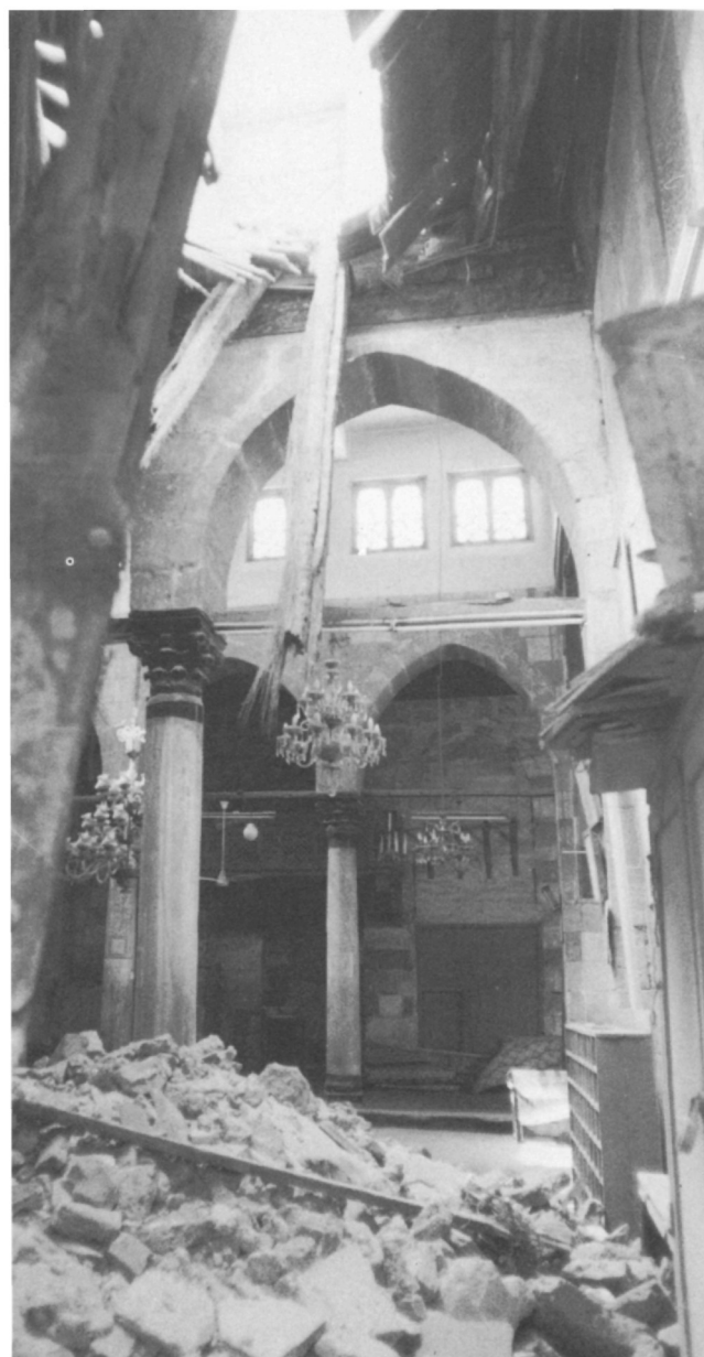
Figure 2.58. Damage to the mosque of al-Tashtushi in the Cairo earthquake of 12 October 1992 (photo: M. Sobaih).
