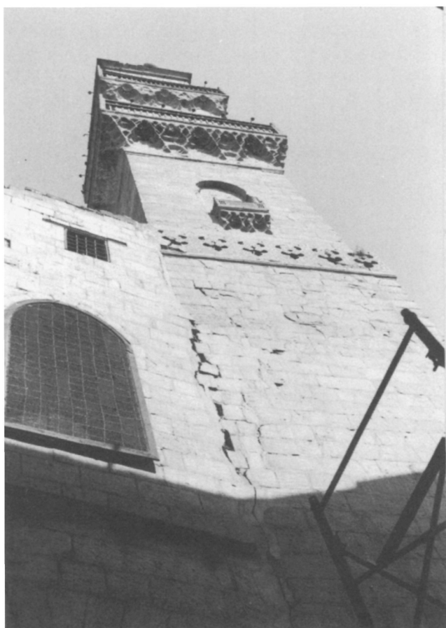
Figure 2.57. Mosque of Sultan al-Ghauri, damaged in the earthquake of 12 October 1992; the walls were already badly cracked before the earthquake (EERI, 1992) (photo: M. Sobaih).
