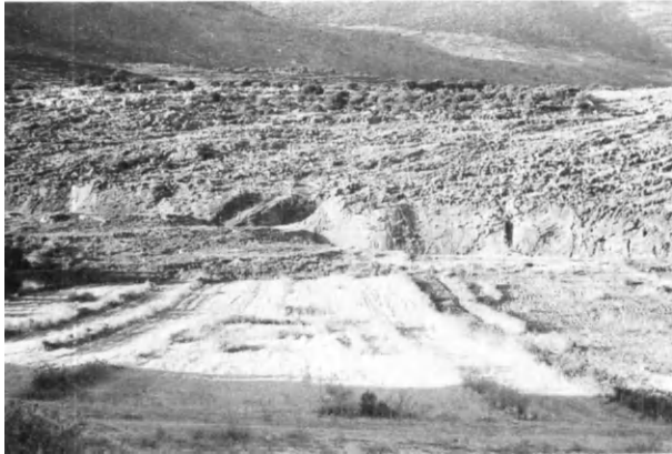
FIGURE 2.77. Fault scarp of the active Bet Kerem Fault, which separates the Lower from the Upper Galilee and extends west to the northern boundary of the Zevulun Valley Rift.
