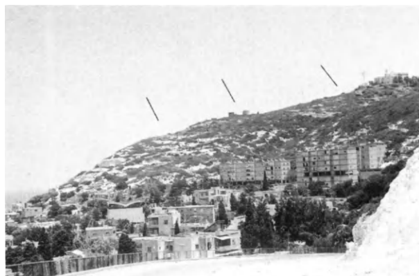
FIGURE 5.22. Abrasion plates, developed on Cenomanian rocks near Haifa. The 110-m (Stella Maris) plate is in the upper righthand corner, where the lighthouse was built. The 80-m plate (Prosper's Tomb) is under the circular building, approximately at the middle of the slope. The 60-m plate is further down.
