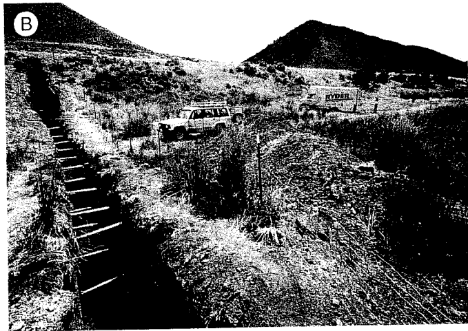
Figure 2.10 Photographs of various types of trenches. (A) Excavating a trench across an 8-m-high normal fault scarp. Eastern Bear lake fault zone, Utah-Idaho (McCalpin, 1993). (B) The finished trench from photograph A, extended well out onto the downthrown block. Supports in trench are hydraulic aluminum shores. (C) Aerial view of stepped bulldozer trench at the Point Conception liquefied natural gas facility. (D) Close-up of benched trench at Point Conception; note persons at far left for scale. (Photographs C and D courtesy of T. K. Rockwell.)
