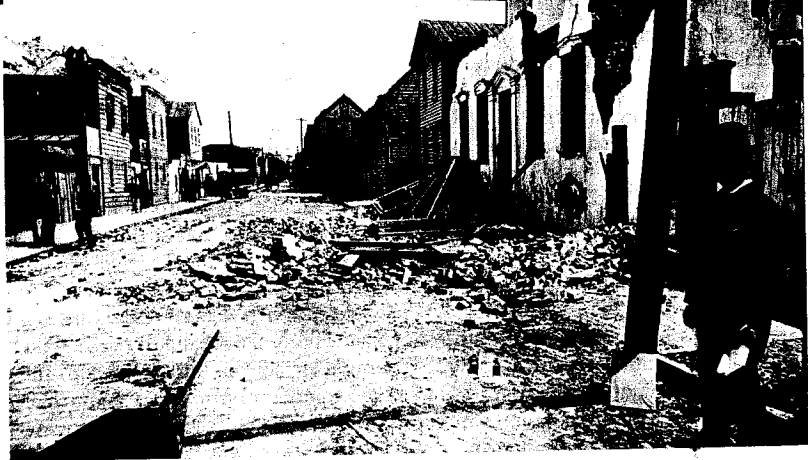
Damage in Charleston, South Carolina, from the earthquake of August 31, 1886. This earthquake is the largest ever reported in the eastern region of the United States. [Courtesy of J. K. Hillers, USGS.]
