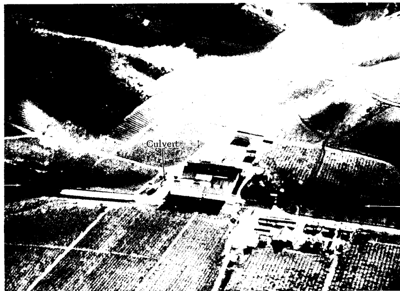
Figure 5.15 Aerial photograph of the Cienega winery built across the San Andreas fault near Hollister, California. The fault (indicated by the horizontal arrows) can be seen extending from left to right, through the culvert on the left (south) side of the winery building and through the building itself. [Courtesy of D. Tocher.]
