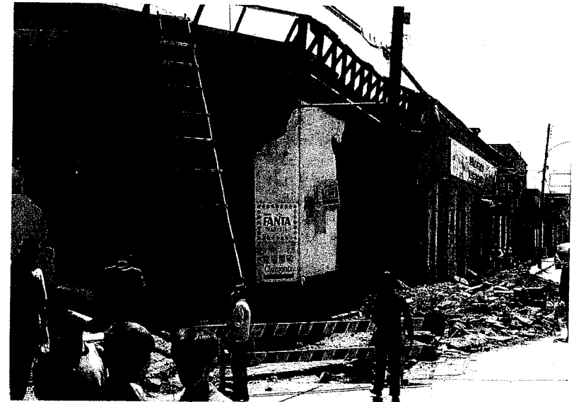
Figure 11.3 Damage to timber frame structures, Melipilla, Chile, in the 1985 earthquake. [Photo by Bruce A. Bolt.]
