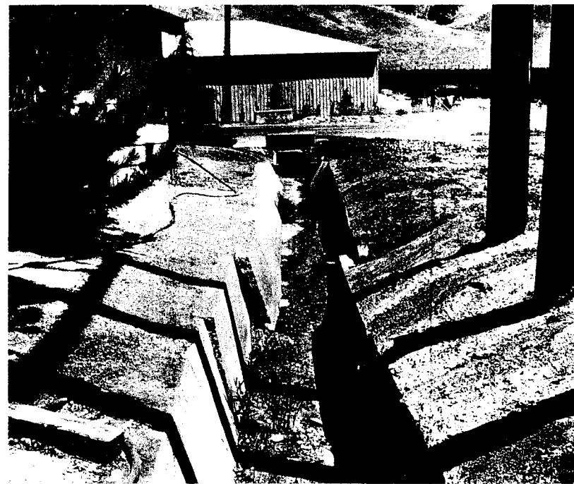
Figure 5.16 Offset of the concrete drainage culvert by slow fault slip along the San Andreas fault at the Cienega winery. This amount of offset has taken place in the course of 20 years. [Courtesy of W. Marion.]
