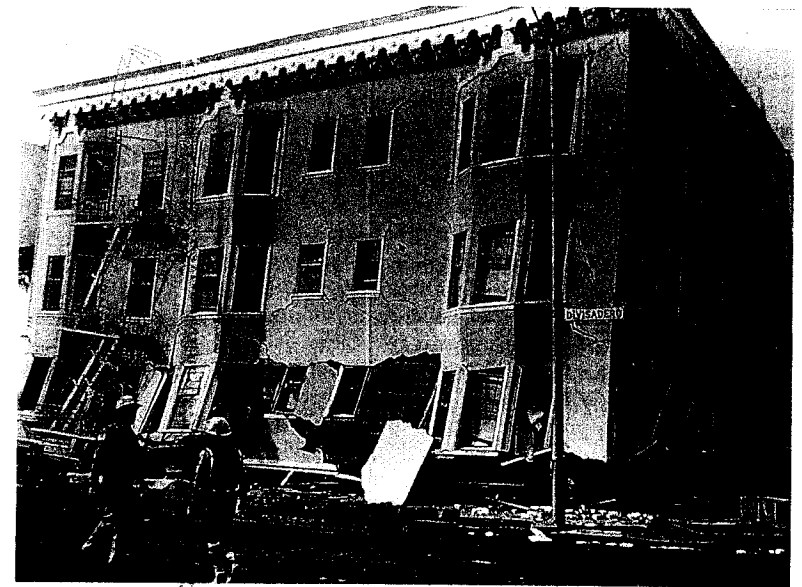
Figure 1.5 Collapse of a four-story timber-frame apartment in the Marina district of San Francisco on October 17, 1989. [Courtesy of S. Mahin.]
