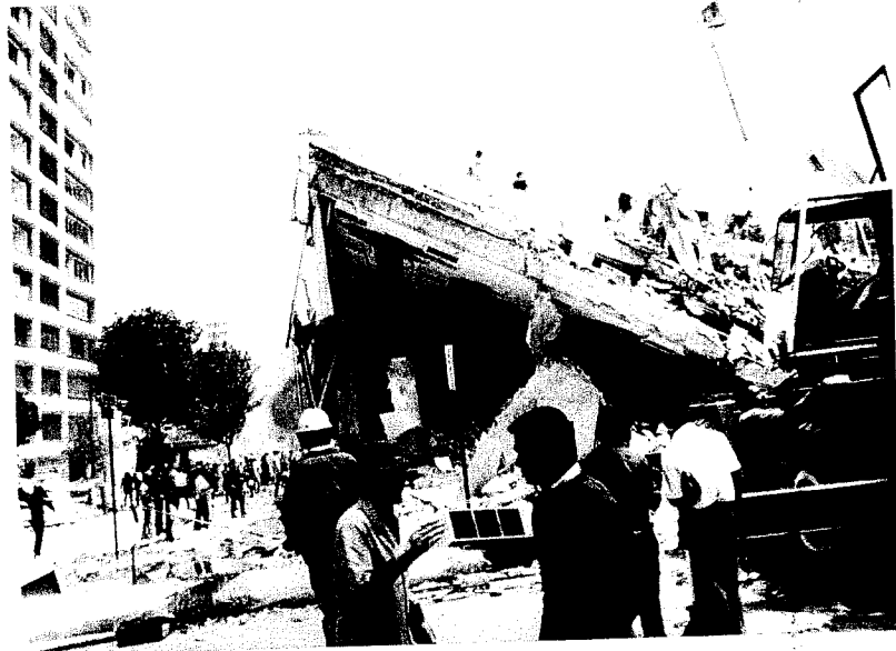
Figure 12.6 Removal of debris from a collapsed reinforced concrete building in the Lake Texcoco zone of Mexico City, September 1985. [Photo by V. V. Bertero.]
