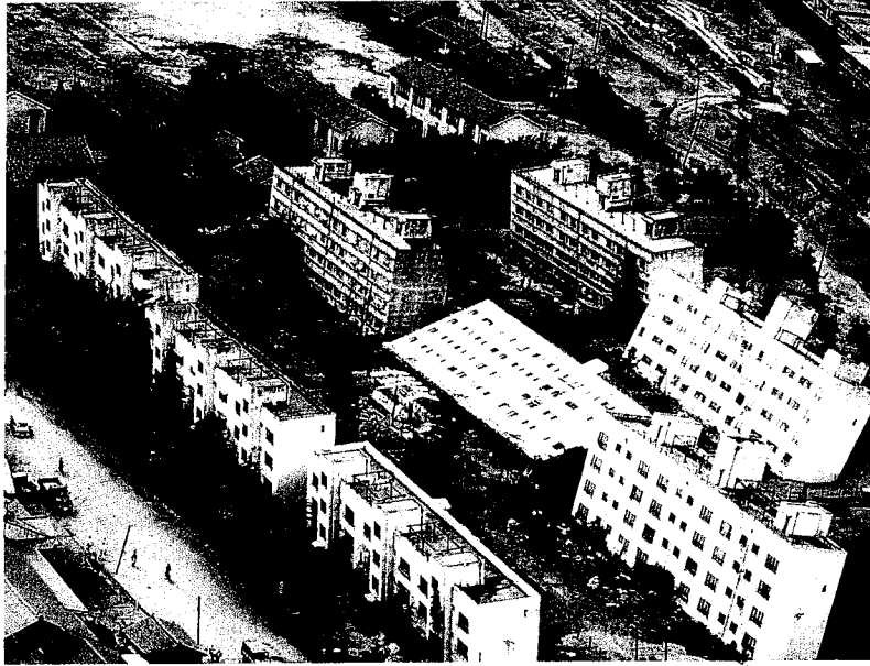
Figure 11.2 An example from the Niigata earthquake of June 16, 1964 in Japan of liquefaction in the foundation sandy soil under apartment buildings. [Courtesy Takeshi Minakami, University of Tokyo, Japan.]
