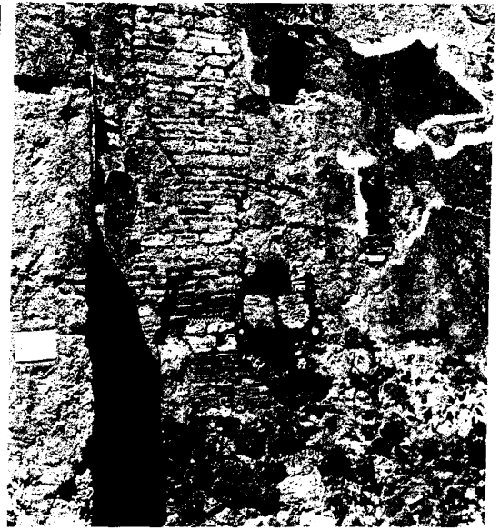
Pompeii. A large fissure in an opus incertum wall, which was filled in after the 62 A.D. earthquake using terracotta materials (tiles and bricks) and rectangular stones. The building can be found in the plan of the city at VI,7,5.
