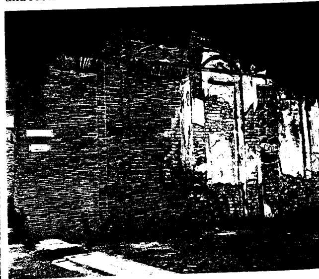
Pompeii. South-west corner of the Building of Eumachia, showing the join between the façade, which was destroyed in the earthquake and rebuilt in brick, and the earlier masonry.
