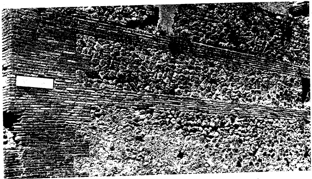
Pompeii. Masonry built after the 62 A.D. earthquake, using opus incertum stones recovered from the ruins, along with regular areas of brickwork.
