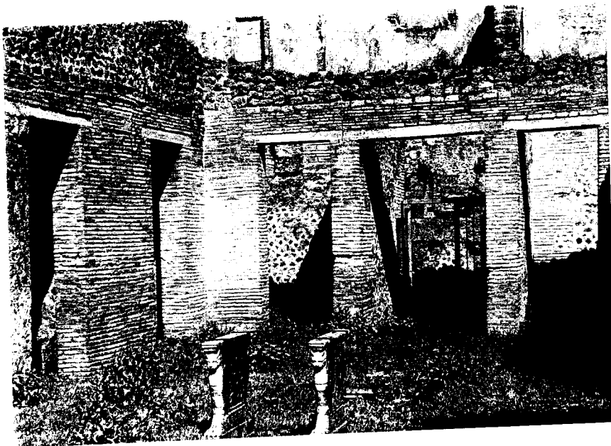
Pompeii. Atrium of the House of Caius Vibius (see city plan VII,2,18), rebuilt after the earthquake of 62, in brick and opus incertum (photo J.-P.Adam).
