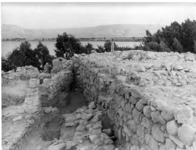
Figure 3.12 Late EB III Wall C at Tel Bet Yerah (Bar-Adon excavations of 1952), looking east. Israel Antiquities Authority archives.
