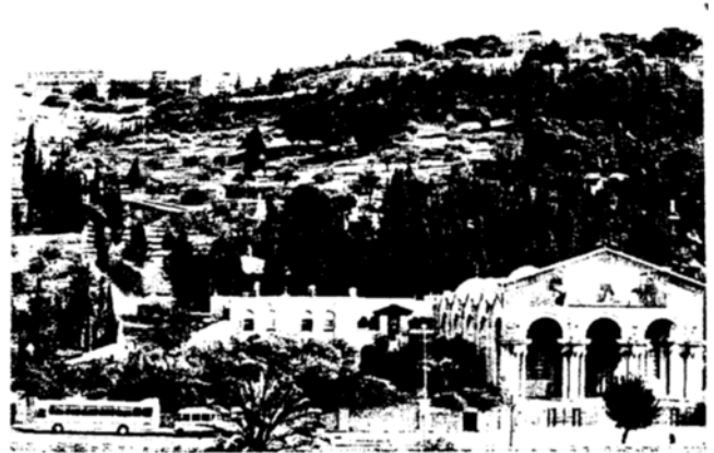
Figure 2. The old landslide in the Mount of Olives. The area clear of trees above the Gethsemane church is the slide unit. Immediately above it, partly hidden behind the trees, is the main scarp ( large arrow ). Younger, smaller scarps can be seen in the left portion of the main slide unit ( small arrow ).
