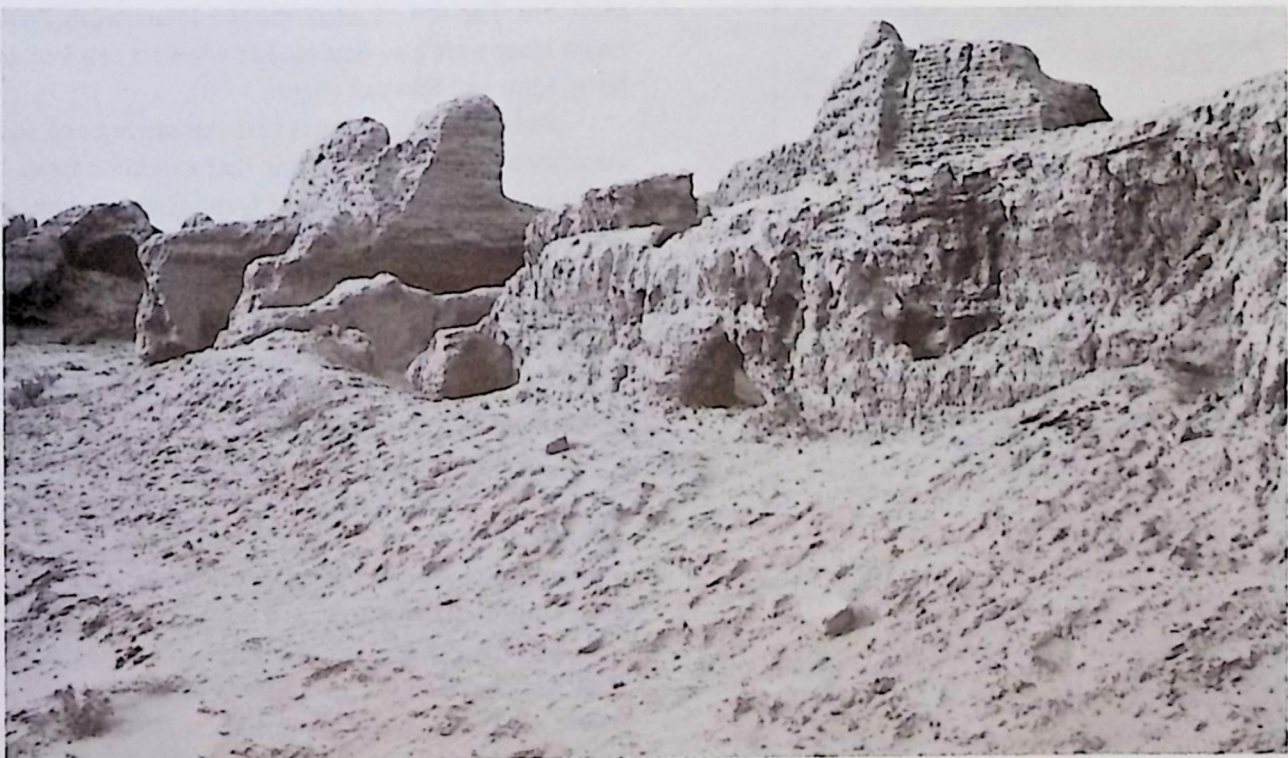
Plate 13. Ruins of the settlement of 'Aliabad Mulla 'Ali Riza, near Buhabad, abandoned after the earthquake of 1933.
