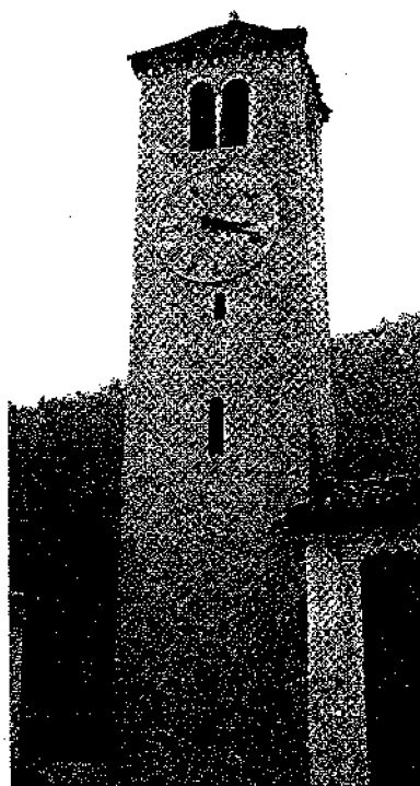
figg. 17 and 18 Costozza (Vicenza), left: bell-tower of the church of S.Mauro; above: inscription on the bell-tower. The earthquakes of 1117, 1222 and 1348 are explicitly recorded. The plaster now in place has covered over the masonry of the various stages of reconstruction and repair of the bell-tower.
