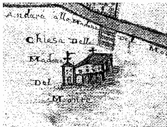
fig. 116 Bologna: the church of the Madonna del Monte (detail from an early 17th century map, now in the Archivio dell'Opera Pia dei Poveri Vergognosi). The church and its bell-tower were badly damaged in the earthquake of 20 December 1455. They stood on top of the nearest low hill to the plain in which Bologna is situated. The church was visited by pilgrims for many centuries. Its remains were enclosed within Villa Aldini at the beginning of the 19th century.
